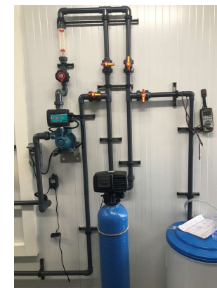
Adsorption with zeolites column
