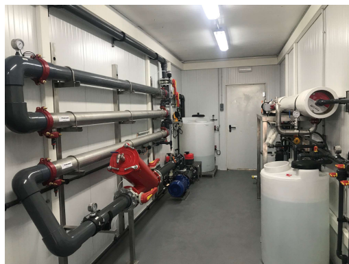
UF unit (left) and RO unit (right)
