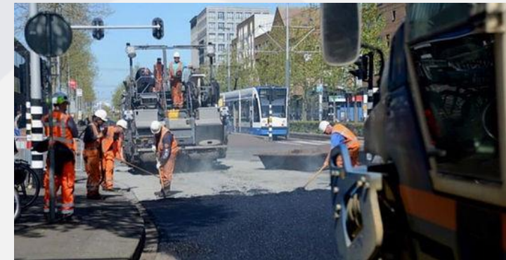
Road constructor KWS uses recycled toilet paper to improve asphalt pavement in Amsterdam
