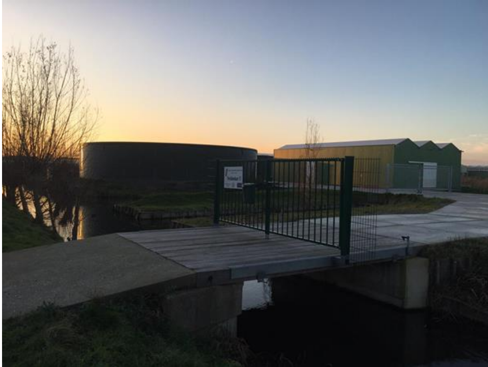
Fig. 5 De Vlot wastewater treatment plant facility
