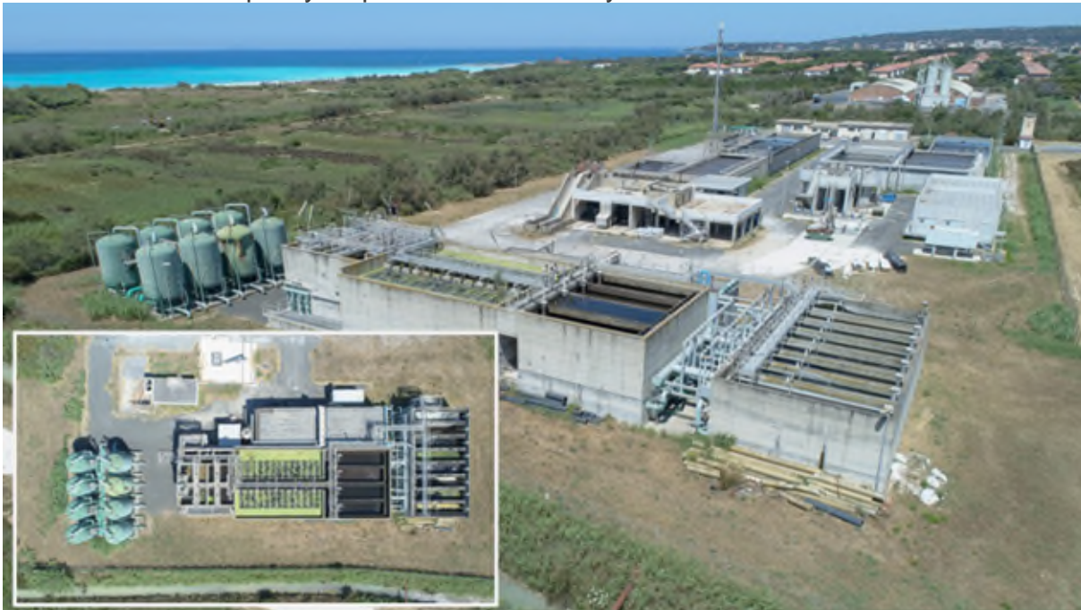
Figure 28. ARETUSA WRP in Rosignano WWTP Area.
