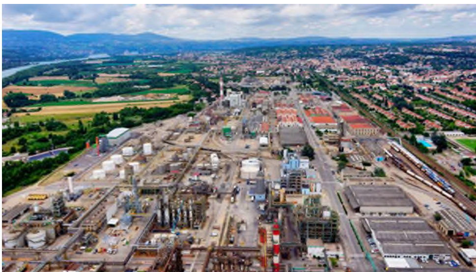
Figure 112. The Roches-Roussillon chemical platform.
