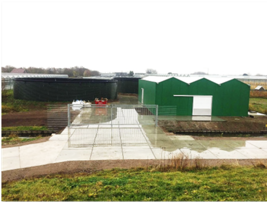
Figure 18. Treatment plant De Vlot.
